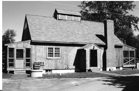
Newly completed Sugar House
