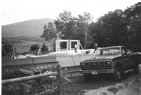
Construction of The English Cottage
